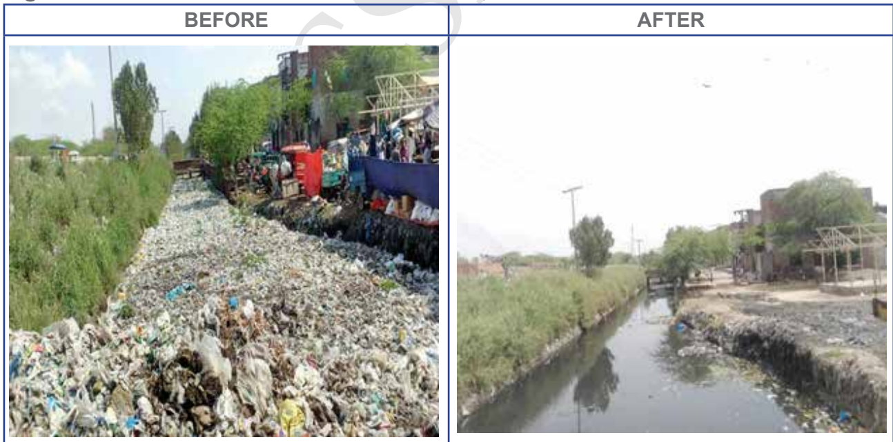
Figure 2: CHANNEL 03 AT NARWALA ROAD, FAISLABAD CITY
